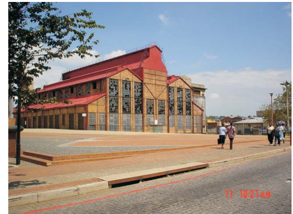
Fig 71. View to Turbine Hall from West Street.
