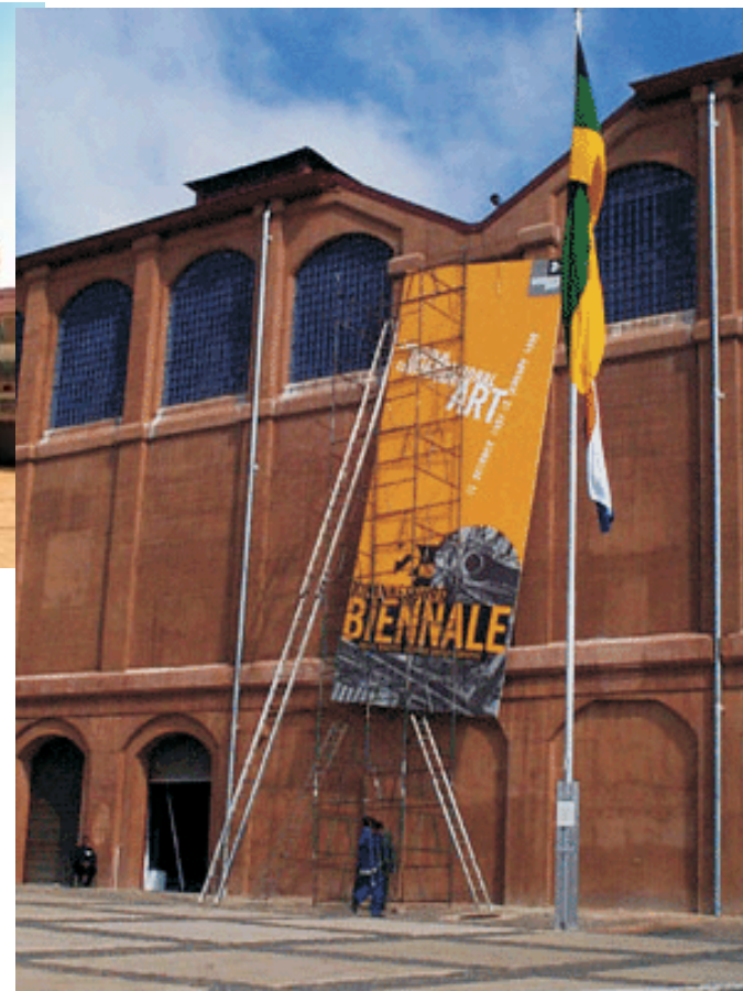
Fig 74. The Electric Workshop.
