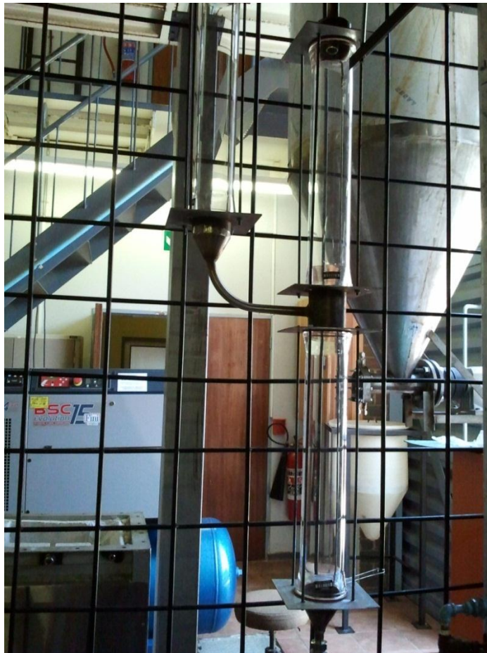
Figure 7.9: Physical construction of quencher section
