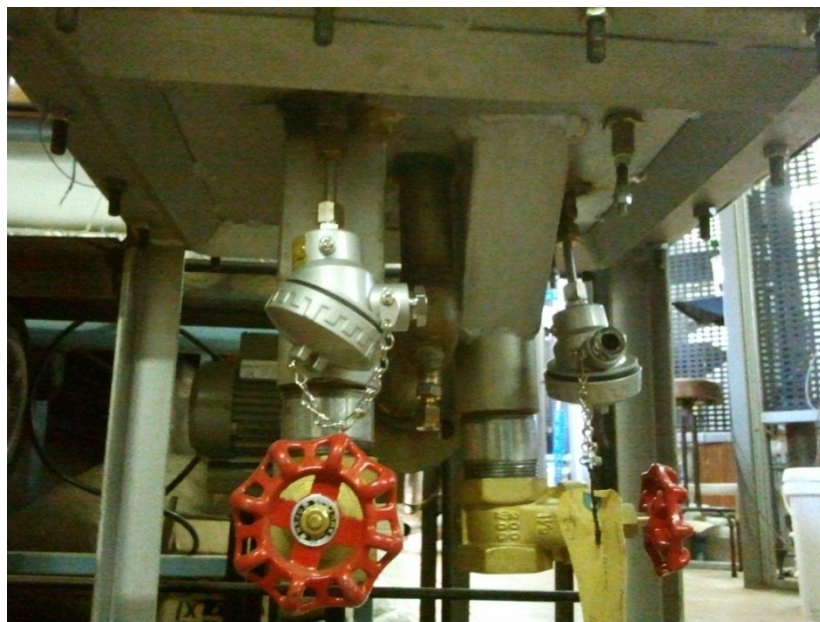
Figure 7.3: Bottom plate and solids outlet on the combustion fluidised bed
