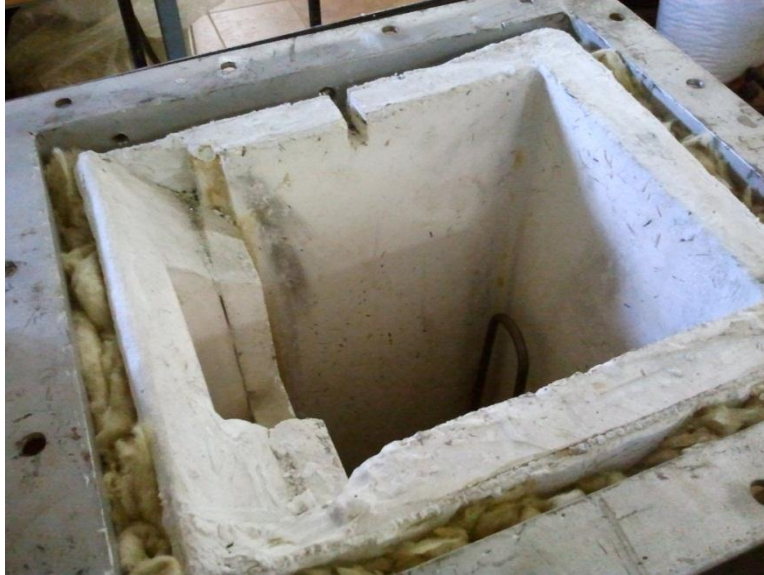
Figure 7.4: Refractory and insulating wool layers in the combustion fluidised bed
