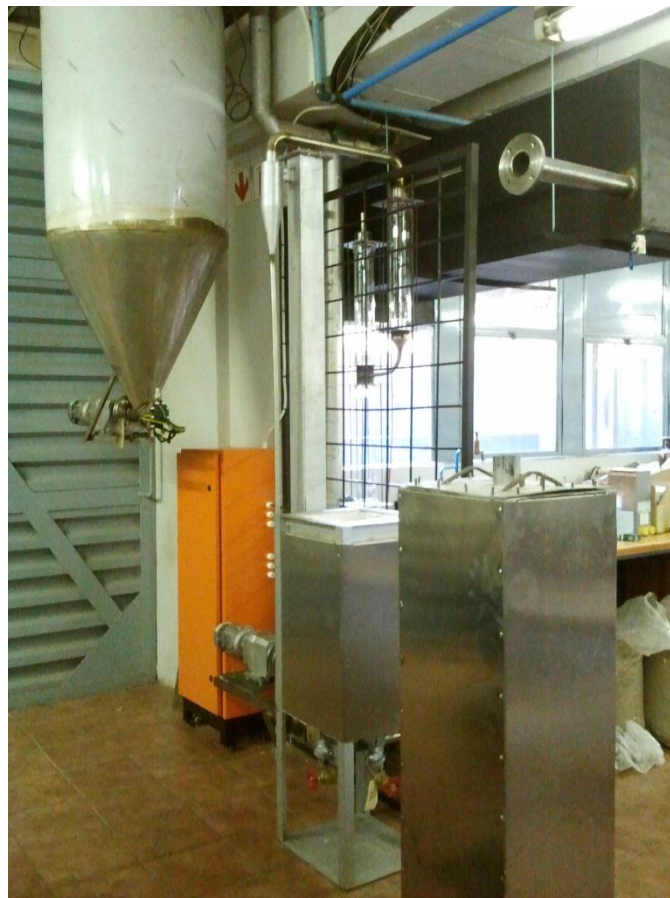
Figure 7.1: Physical construction of the pilot-scale system
