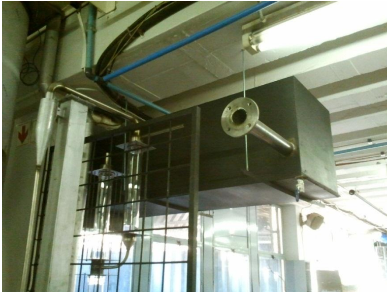
Figure 7.10: Physical construction of extraction box
