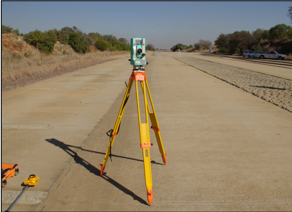
Figure 41: Ground control points surveyed using a Total Station.
