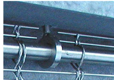
Fig. 8.8. Detail of rod eyebolt connection
