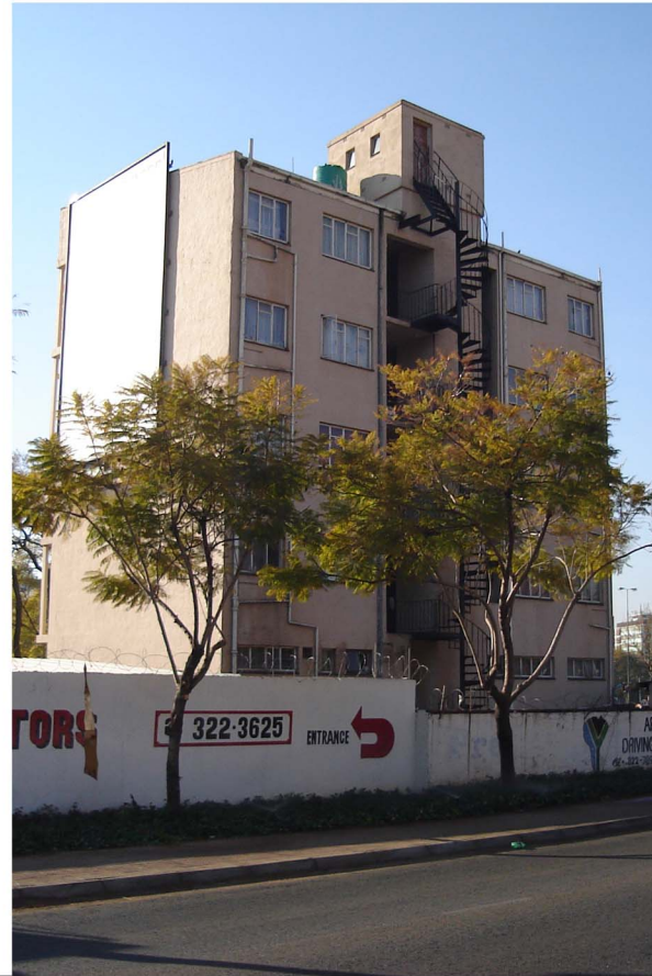
Fig. 7.20. The view from Skinner Street revealing the rows of windows on the back facade
