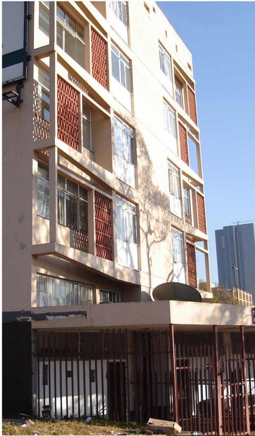
Fig. 7.19. The Ribbon Window and Free Facade 'with 'Brise Soleil' Screens
