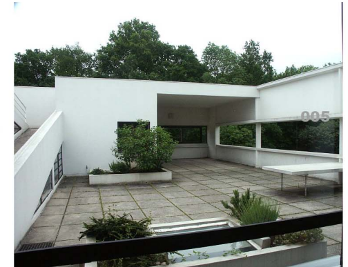
Fig. 5.12. A view of the terrace from the living room
