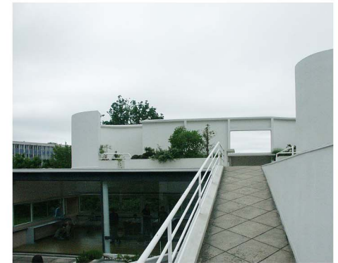
Fig. 5.17. The framed view at the end of the ramp
