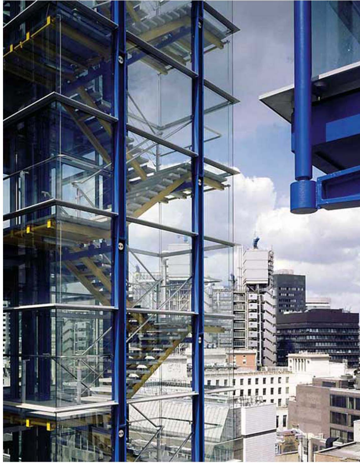
Fig. 5.47. The glazed service towers are constructed of light tubular steel frameworks
