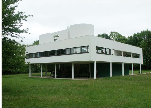
Fig. 5.1. The Villa Savoye, framed by the surrounding landscape
