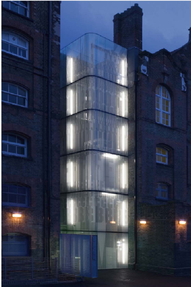
Fig. 5.48. The new entrance and lift shaft of the Victorian Credon Centre
