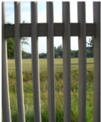
Figure 82: The palisade fence and open buffer zone are not a welcoming site (Author, 2008)
