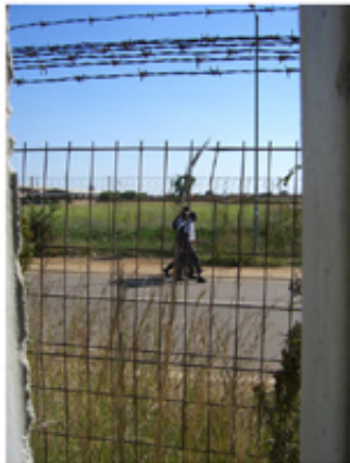
Figure 81: Intimidating double wire + palisade fence surrounding the campus (Author, 2008)
