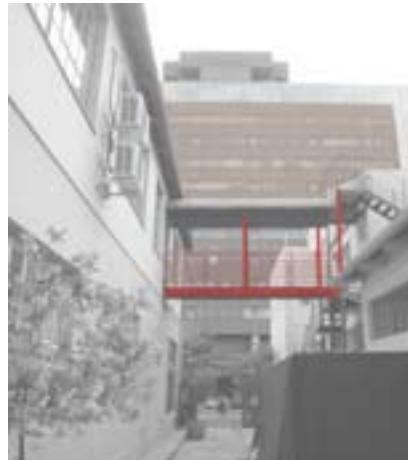
Fig. 4.5 Alley between buildings.
