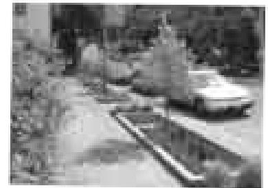
Fig. 6.139 A wide street section accommodates stormwater treatment.
