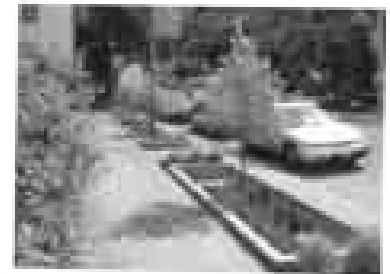
Fig. 6.139 A wide street section accommodates stormwater treatment.
