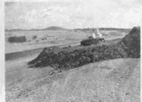
Fig.6.33 Distribution of topsoil.
