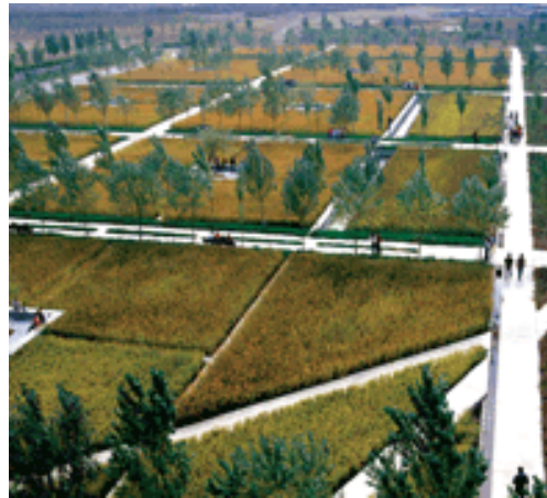
Fig. 4.21 Aerial view of Shenyang Architectural University.
