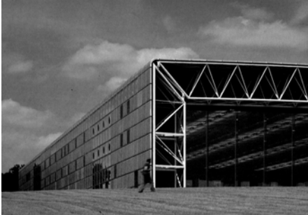
Sainsbury Centre from the south showing top lighting from strips of glazed panels.
