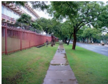
Figure 4.6: Minnaar Street pedestrian walkway in front of new Fire Station; note palisade fence and walkway can be widened
