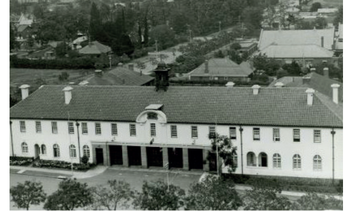
Figure 4.14: The Old Fire Station building with the original clay tile roof (Source: Archive of Department of Architecture, UP)
