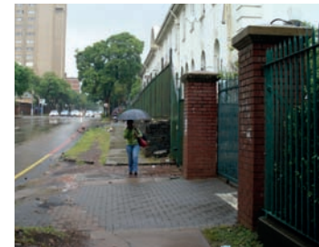
Figure 4.9: Bosman Street; palisade fence and pedestrian walkway uneven and broken
