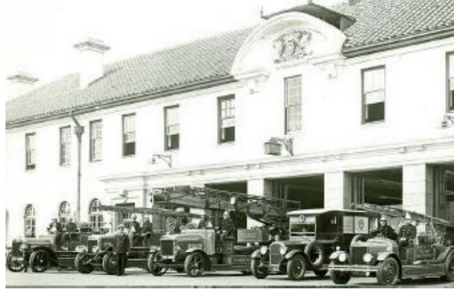
Figure 4.13: The Old Fire Station building in use (Source: Archive of Department of Architecture, UP)
