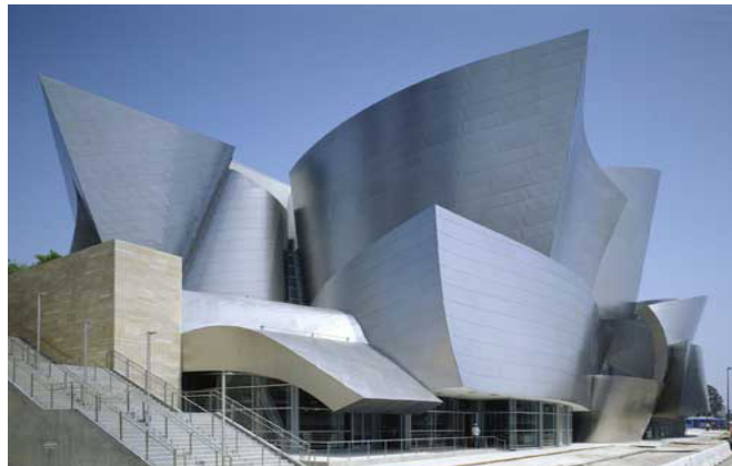
ILLUS. 60 Walt Disney Auditorium by Frank Gehry ( arcspace, 2011) (available at http://www.arcspace.com/architects/gehry/disney2/ )
