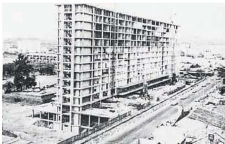
fig. 3.13 Munitoria under construction.
