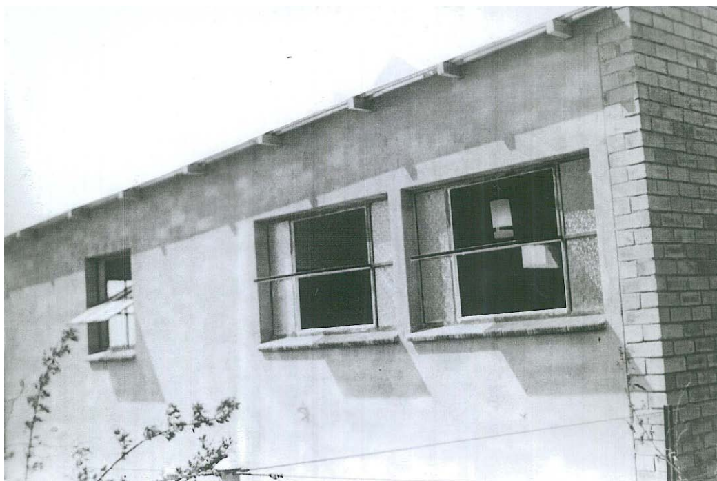
The first church building in Laudium: A garage built on the Evangelist's premises
