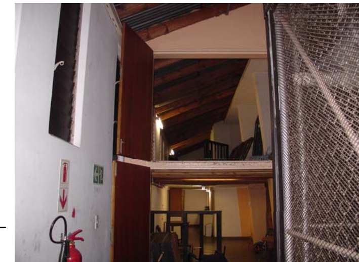
Figure 2.1.25: Interior view of the extension used as storage for props and lighting
