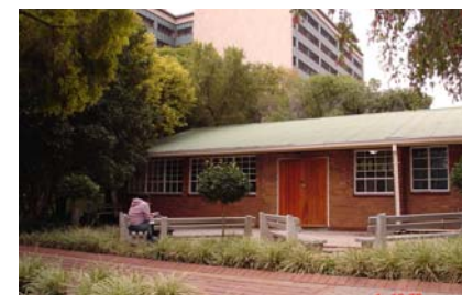
Figure 2.1.32: Photograph of the exterior of Die Bok
