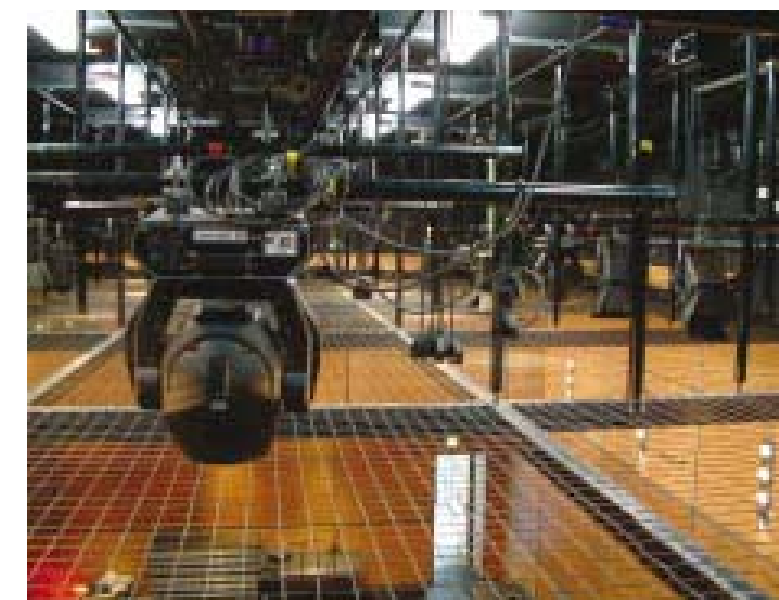
Figure 6.1.6: This system, a 15 x 8m containment Frame, features an integral support structure complete with hangers and lighting grid, and is installed on the first floor of a Georgian villa that is now known as CCA Glasgow. Tension wire grid platforms are woven from stainless or galvanized steel wire rope
