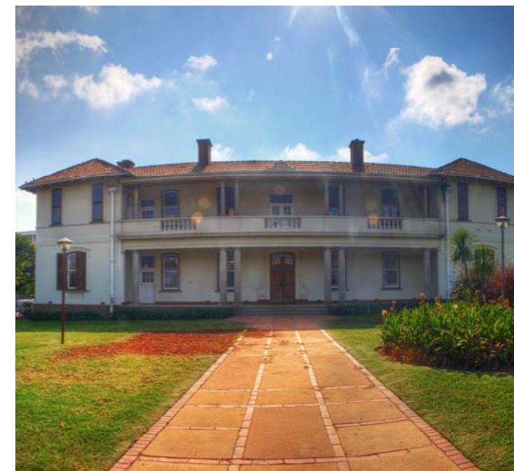
Figure 2.1.6: Panoramic photo of the Drama Building from Lynwood Road, Misra, S May 2008
