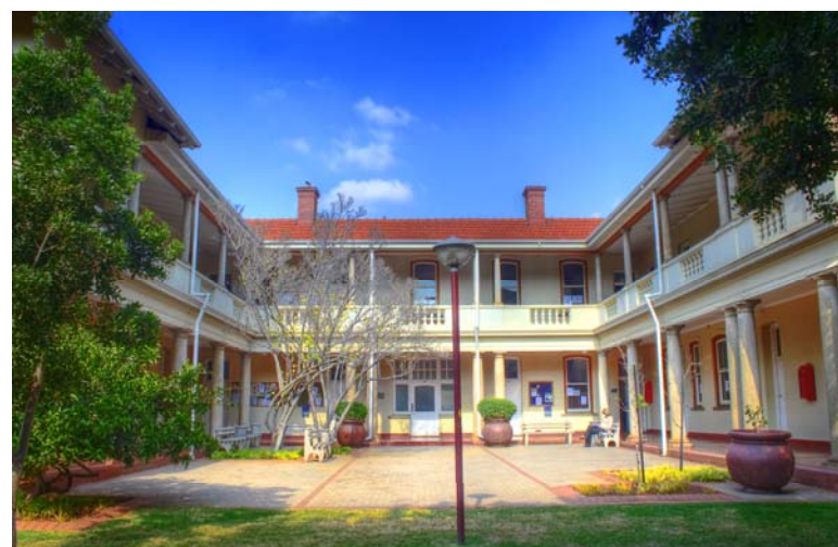
Figure 2.1.9: Panoramic view of the courtyard to the Drama Building (old CBC), by Misra, S, May 2008
