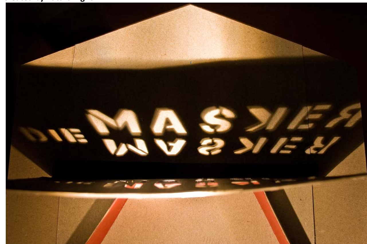
Figure 5.1.20: Photograph of the lighting effect of the entrance canopy during at night for performances. Silhouette created by lighting from below light.
