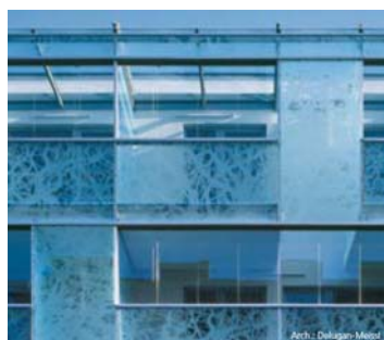
Figure 6.1.10: Screen printed glazing: Double glazed screen printed glass in anodized aluminium window frames Laminated safety glass of 4mm with images screen printed. External windows to be double glazed. Maximum sizes: 1500mm x 3000mm. Utilized in the glazed envelope of the extension to Die Masker staircase seen from the square.
