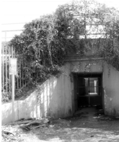
FIG 39: Existing entrance: inactive.
