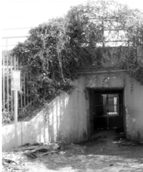
FIG 39: Existing entrance: inactive.
