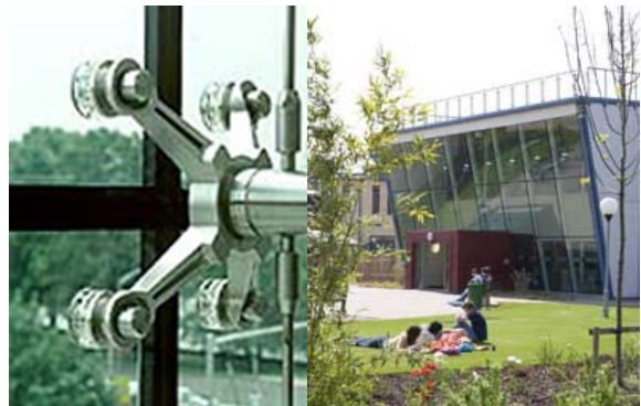
Figure 7.55: Pilkingtons planar glazing system
