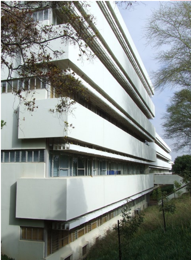
Figure 2.39: Photograph of Administration Northern fa-
