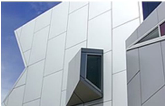
Figure 7.57: Composite aluminium cladding panels
