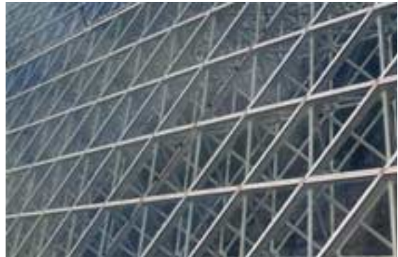
Figure 7.54: Space frame structure
