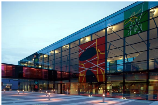
Figure 5.26: Facade of Building
