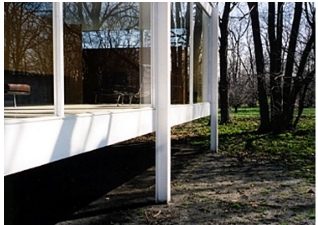
Figure 4.2: Mies van der Rohe`s Farnsworth house
