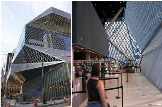
Figure 7 51: OMA's Seattle library steel structure
