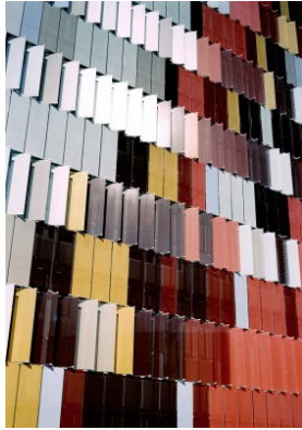
Figure 5.8: Glass Louvre Facade
