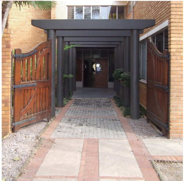
Figure 2.37: Photograph of Visual Arts main entrance
