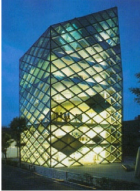
Figure 5.31: Exterior night time view of prada store
