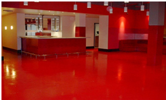
Figure 7.60: Epoxy resin floor finish
