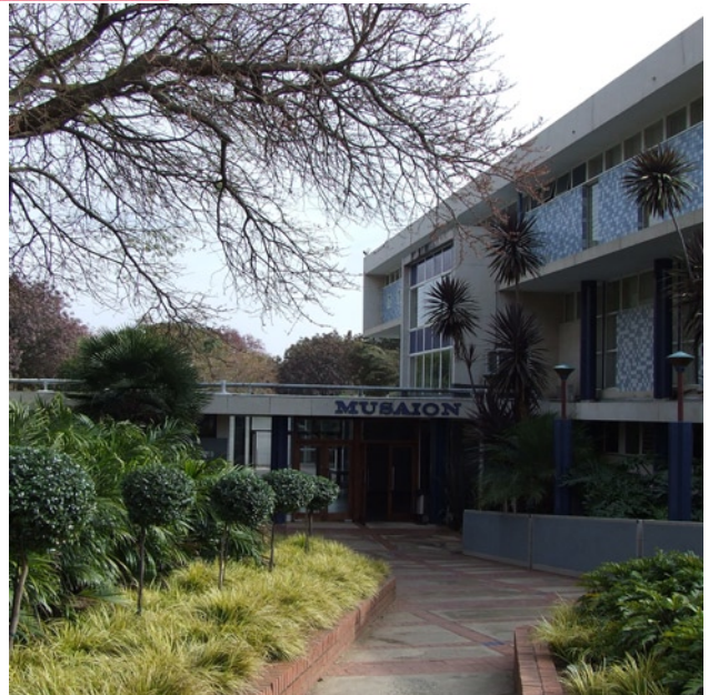
Figure 2.43: Photograph of Musaion main entrance
