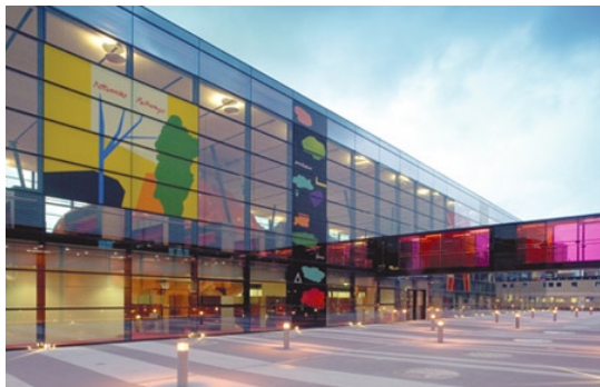
Figure 5.28: Connecting bridge of building
