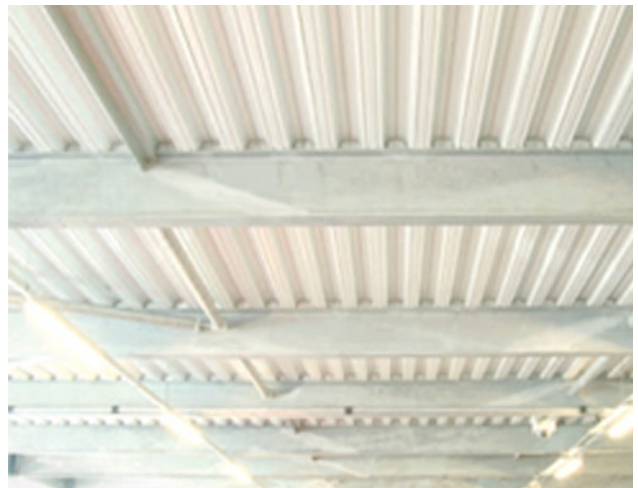
Figure 7.12: Photograph of floor before finish
