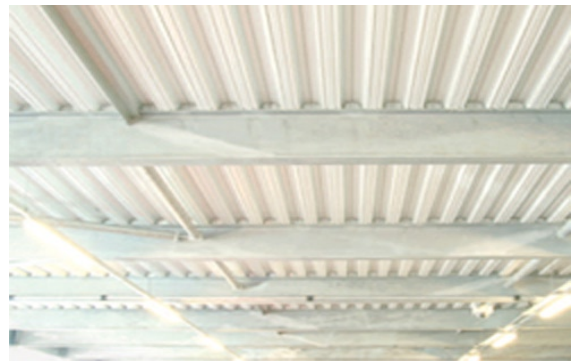
Figure 7.53: Composite floor slab
