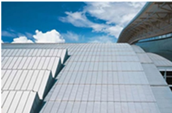
Figure 7.58: Zinc standing seam roof cladding
