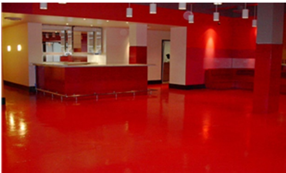
Figure 7.60: Epoxy resin floor finish
