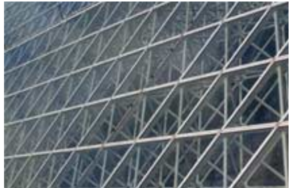
Figure 7.54: Space frame structure
