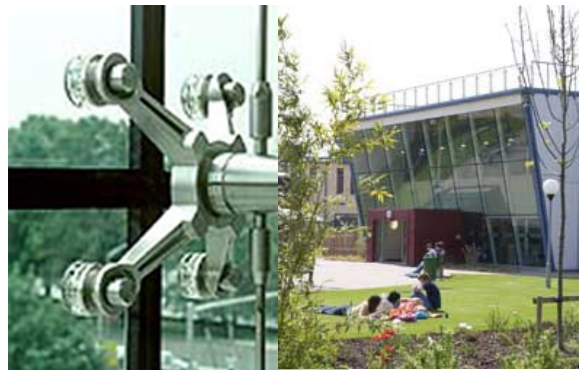
Figure 7.55: Pilkingtons planar glazing system
