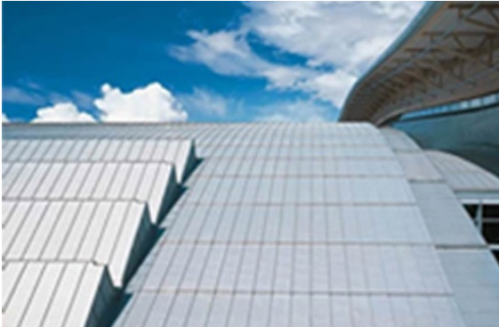
Figure 7.58: Zinc standing seam roof cladding
