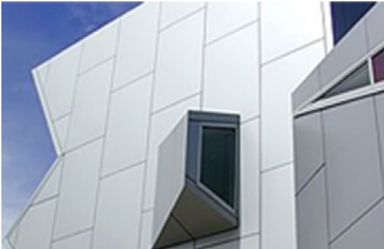
Figure 7.57: Composite aluminium cladding panels
