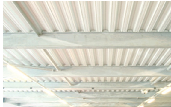
Figure 7.53: Composite floor slab
