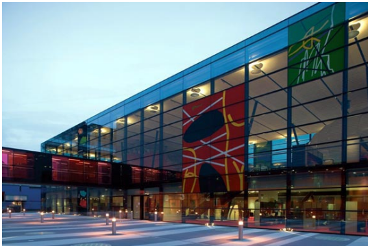
Figure 5.26: Facade of Building
