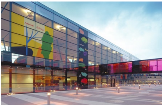
Figure 5.28: Connecting bridge of building
