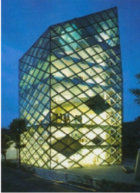
Figure 5.31: Exterior night time view of prada store
