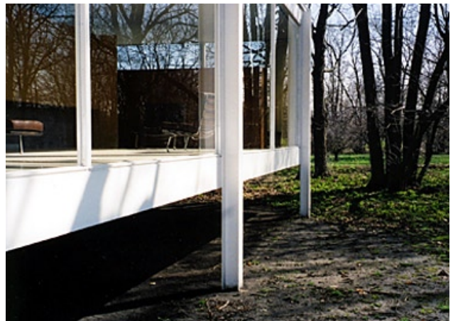
Figure 4.2: Mies van der Rohe`s Farnsworth house
