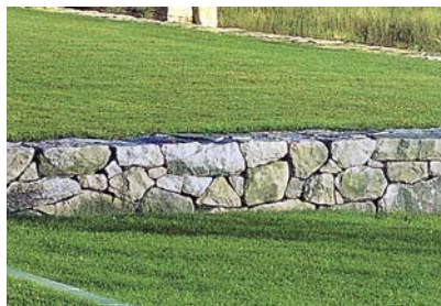
Fig. 9.78: Stone packed retaining wall (Asensio 2005)
