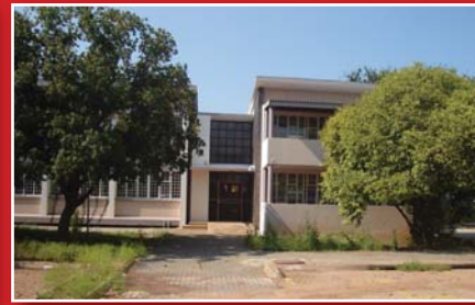
4: Pharmacy (to be demolished)
