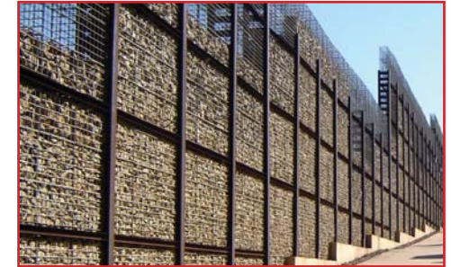
Fig. 9.16: Rock-filled wiremesh and steel structure. (Author, 2008)
