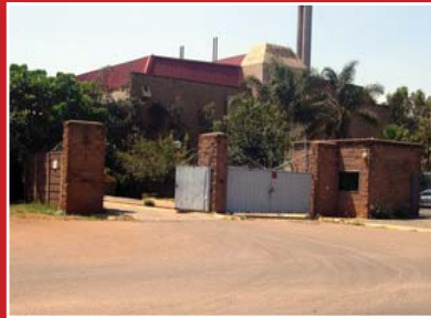
8: Services core buildings (northern elevation)
