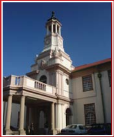
1: Main administration (southern elevation)
