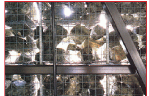
Fig. 9.18: Rock-filled wiremesh and steel structure. (Asensio, 2005)
