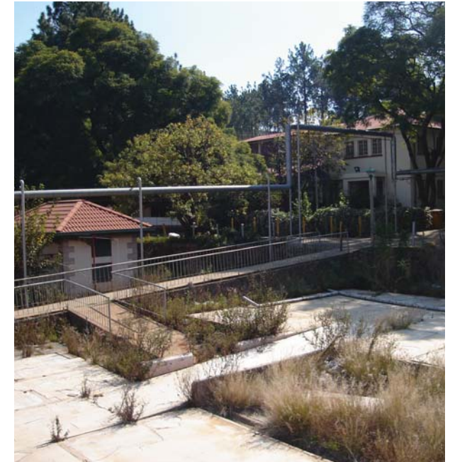
Fig. 3.21: Remains of demolished buildings (2008 and Author, 2008)
