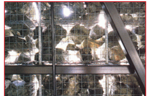
Fig. 9.18: Rock-filled wiremesh and steel structure. (Asensio, 2005)
