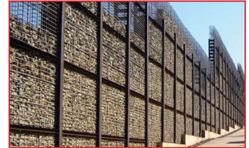
Fig. 9.16: Rock-filled wiremesh and steel structure. (Author, 2008)
