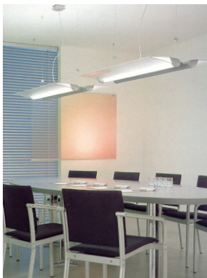
Fig 178. Individual task lighting
