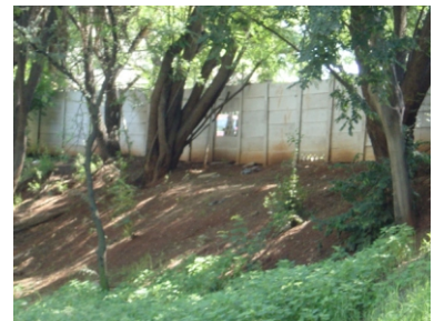
Fig 16. View of wall from Apies River
