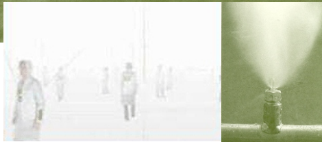
Fig 67. Nozzles used to create fog
