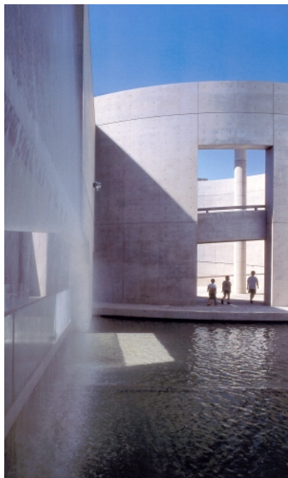
Fig 182. Off-shutter concrete finish
