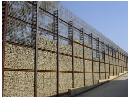
Fig 181. Gabions / Stone walls
