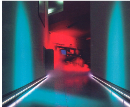
Fig 176. Corridors lighting on floor level
