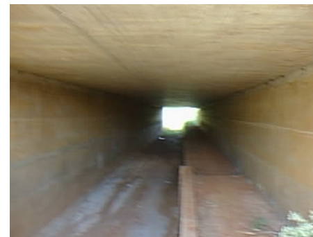
Fig. 12: Inside the Tunnel
