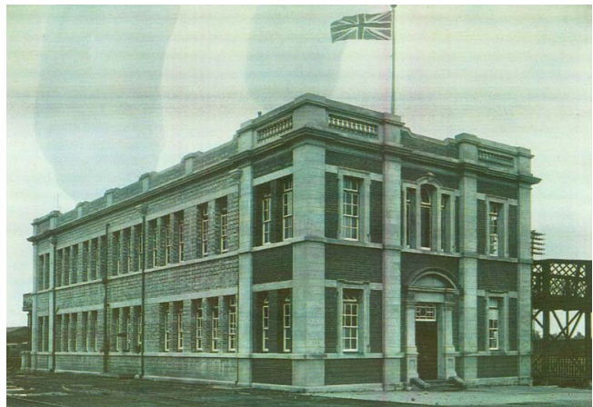
Illus 1.3 Chief Engineer’s Office, 1909 (Bakker, 2002)
