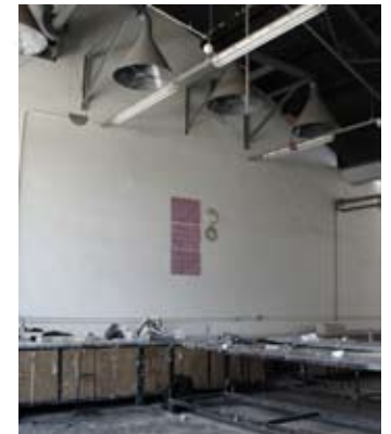
Figure 39: Existing building interior.
