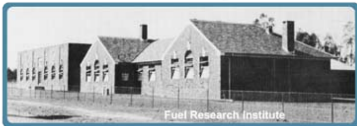
Figure 29: First buildings of the Fuel Research Institute completed in 1933.
