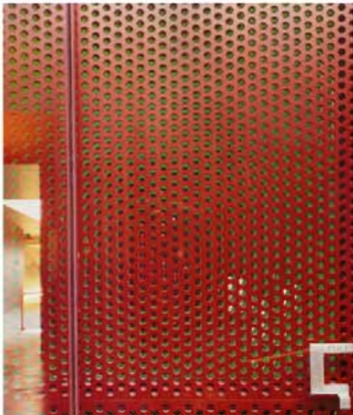
Illus. 128 (left) Cranbrook Institute of Science, Michigan, 1999, Steven Holl Architects. Double layer perforated plywood panels showing the effect the perforated steel plate will have on the eastern facade.(OJEDA ET AL 2003: p.22)
