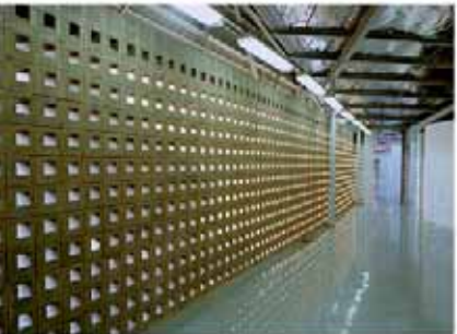
Illus. 56 Photograph of re-facing with custom designed bird proof concrete blocks to enable natural cross ventilation and filtering of northern light. LR Plastics Factory, 2005-2006, Durban, studioMAS and soundspacedesign. (LOW 2007: p.93)
