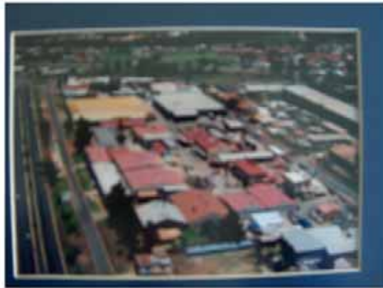
Illus. 62 Aerial Photograph of Plascon Factory, Krugersdorp, South Africa. Unknown architect. (Author 2007)
