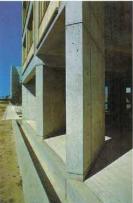
Illus. 123 Salk Institute for Biological Studies, passage under administration offices, La Jolla, California, Louis I. Kahn 8.2.1 CONCRETE
