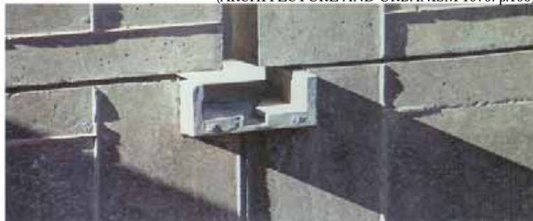
Illus. 114 Salk Institute for Biological Studies, scupper on balcony corridor, La Jolla, California, 1959-1965, Louis I. Kahn. (ARCHITECTURE AND URBANISM 1975: p.195)
