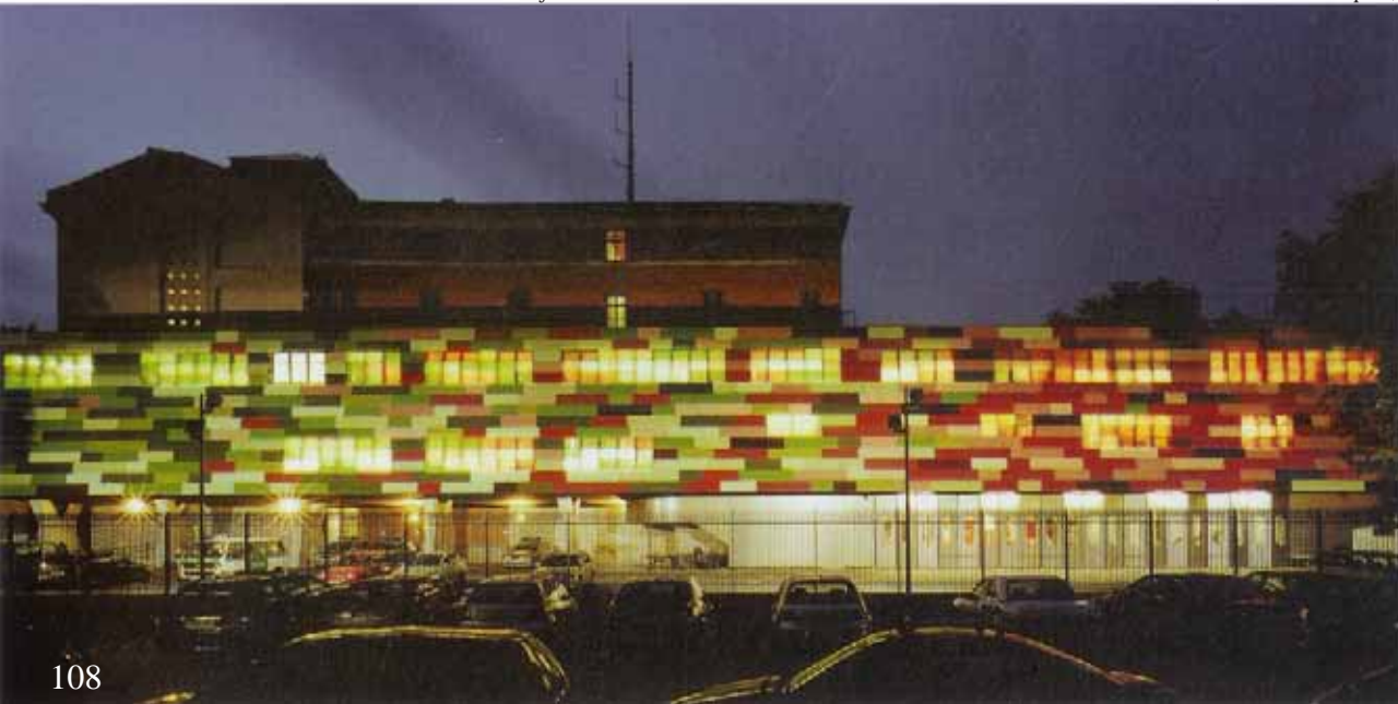
Illus. 116 Fire and Police Station, Berlin, Germany, 2004, Sauerbruch & Hutton.
