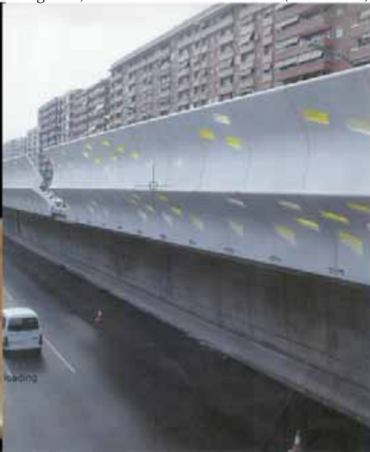
Illus. 50 Photograph of Gran Via Expressway acoustic panels, showing the coloured glass inserted into the concrete skin, Spain, EMBT (Enric Miralles and Benedetta Tagliabue) (EMBT 2007)
