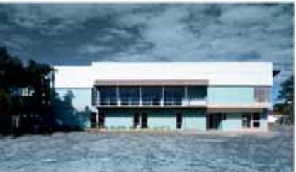
Illus. 54 Photograph of refurbishment of the old Novilon building for the LR Plastics Factory, Durban, 2005-2006, studioMAS and soundspacedesign. (LOW 2007: p.88)
