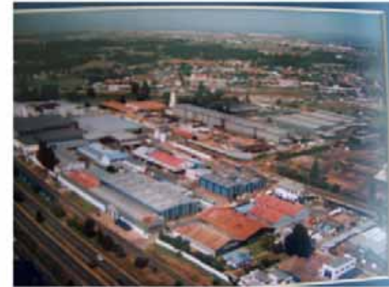
Illus. 64 Aerial Photograph of Plascon Factory, Krugersdorp, South Africa. Unknown architect. (Author 2007)
