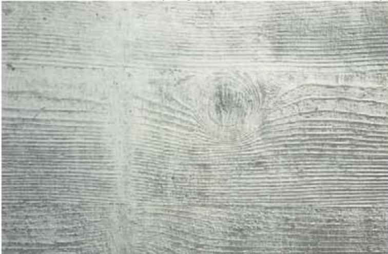
Illus.124 Concrete texture created by rough sawn timber boards.(DEPLAZES 2005: p.57)
