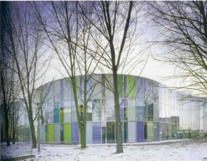
Photonics Centre, Berlin, Germany, 1998, Sauerbruch & Hutton (MOOR 2006: p.34)
