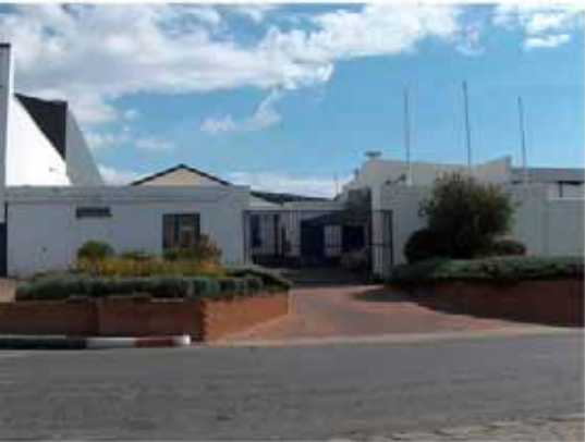
Illus. 61 Exterior view of entrance to Plascon Factory, Krugersdorp, South Africa. Unknown architect. (Author 2007)
