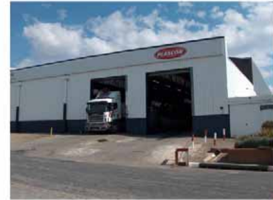
Illus. 66 Exterior view of dispatch area. Plascon Factory, Krugersdorp, South Africa. Unknown architect. (Author 2007)
