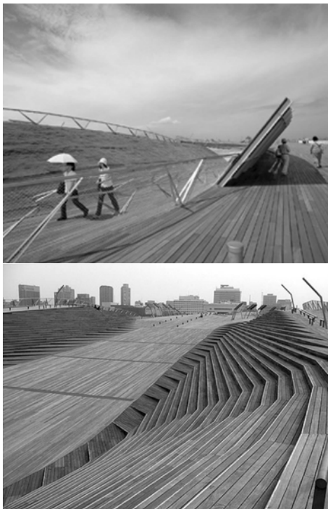
Fig. 115 & 116. Yokohama International Port Terminal (www.foa.net 16 July 2007).
