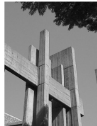
1 Off shutter concrete structure, defining the Entrance - Doxa Deo
