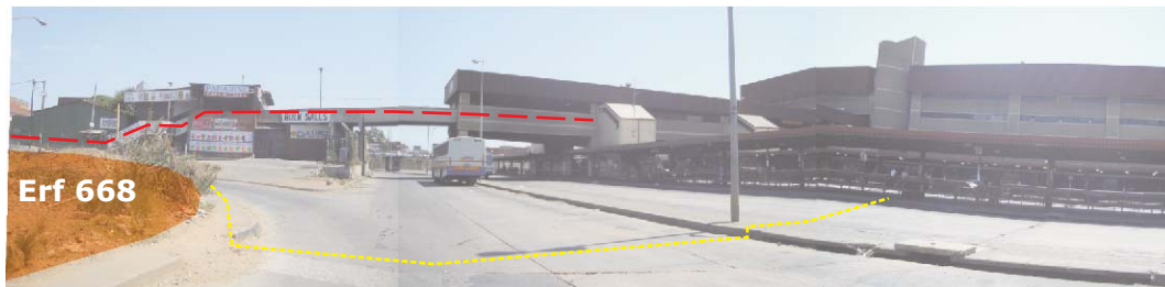
Figure 4.8: View of Belle Ombre train station and access bridge
