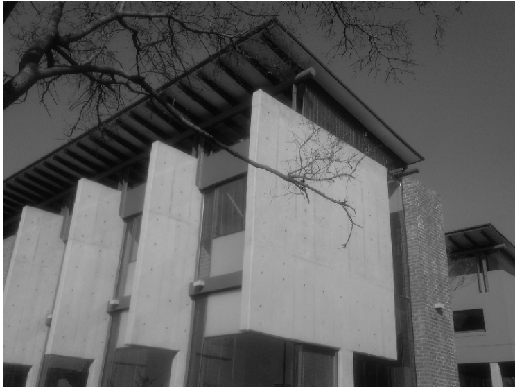
Figure 5.33: Tolplan - concrete fins (Author 2007)
