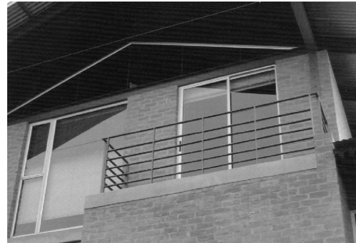
Figure 5.31: House Steyn - balcony detail (Botes 2006: 53)
