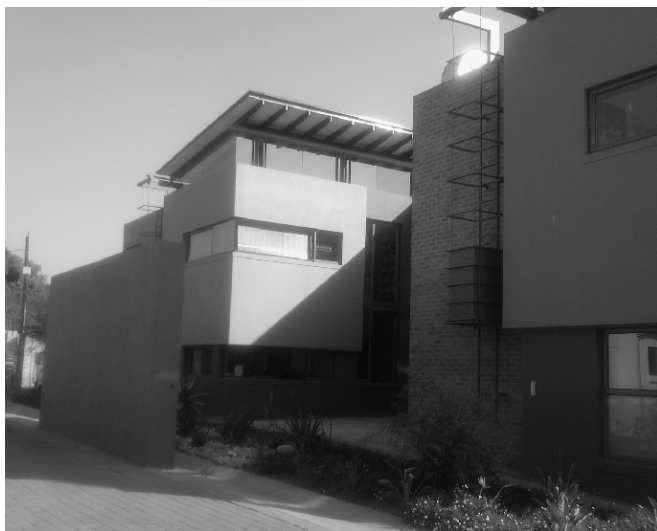
Figure 5.38: Tolplan - Eastern facade with courtyard (Author 2007)
