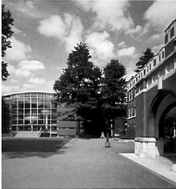
Figure 5.15: Approach to library (Webb 2007: 60 )
