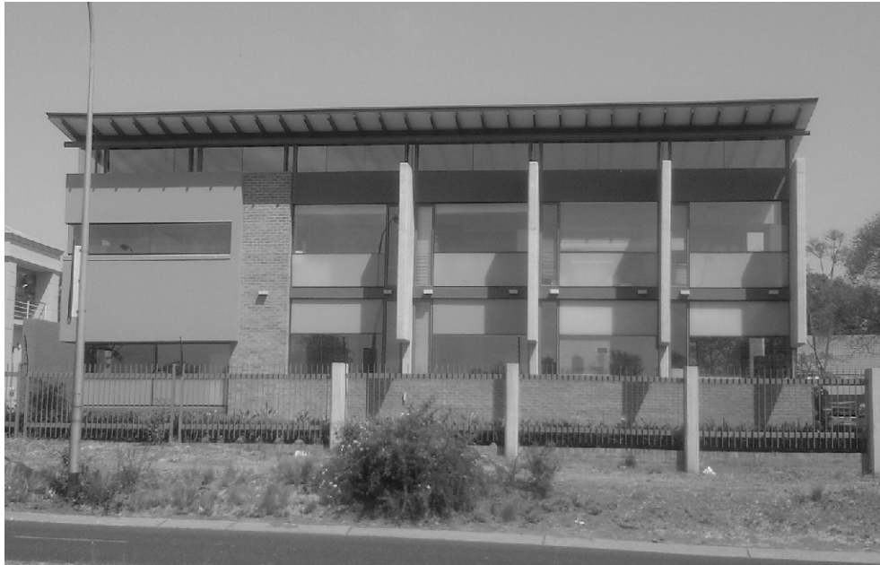
Figure 5.37: Tolplan - front facade from Lynnwood street (Author 2007)
