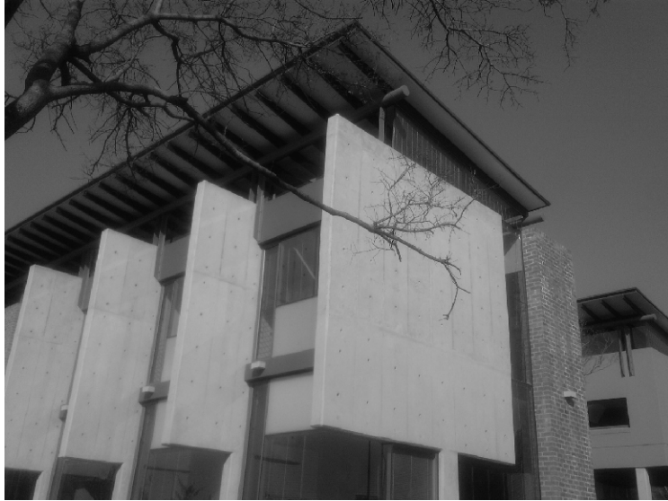
Figure 5.33: Tolplan - concrete fins (Author 2007)
