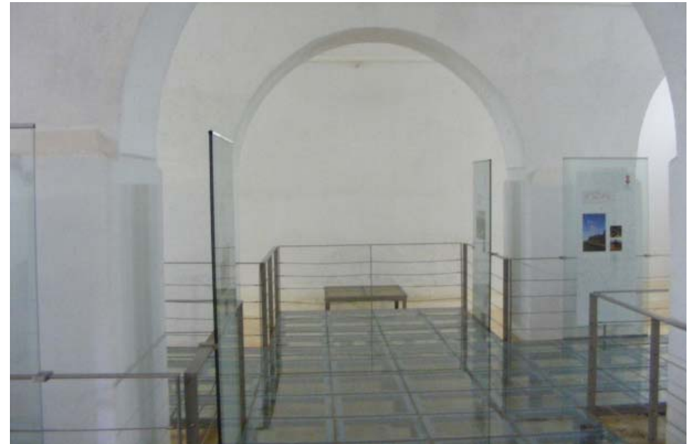
Illus. 61: View within the water reservoir. Elevated glass boardwalks are used to take the visitor inside the reservoir and over the old flooring. The glass ensure a clear view of what goes on underneath. Glass signage is used to communicate the history. (Gryffenberg, 2010)
