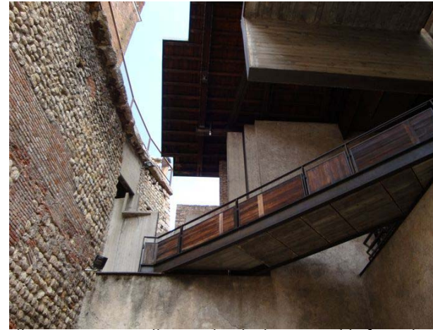
Illus. 49: A new walkway, clearly distinguishable from the old castle. (Anniforscia, 2008)
