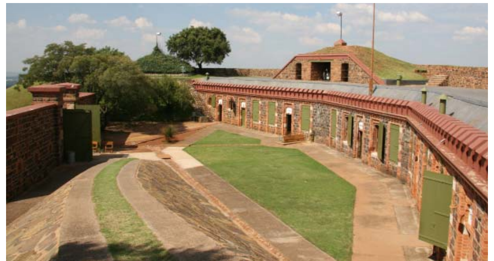
Illus. 39: Example of restoration. Fort Klapperkop (1898), restoration done by Anton van Vollenhoven (Author, 2011)
