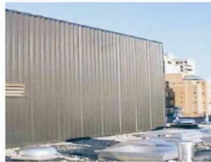
▲ fig7.6 An Example of a Transpired Wall (Brown 2001, p.238)
