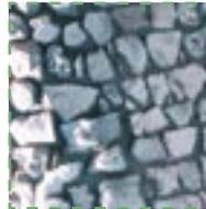
The western wall wrapping around the building, leading to the entrance, is made of a steel mesh frame filled with stone (like gabion walls) through which soft light and air flows freely. Evaporative cooling pools are drained in winter leaving a rock bed. These rock beds are a theme carried throughout the Centre.
