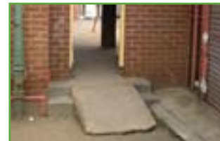
Too steep level change and irregular floor surface
