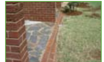
Too steep level change and irregular floor surface
