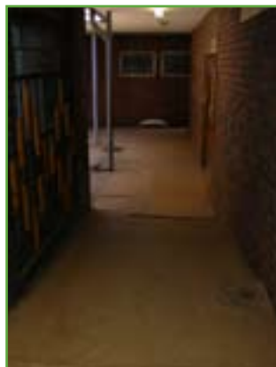
Dangerous space • Steep ramp – collisions can take place against opposite wall • Gully and mat = obstruction • Rainwater is not channelled away and forms puddles
