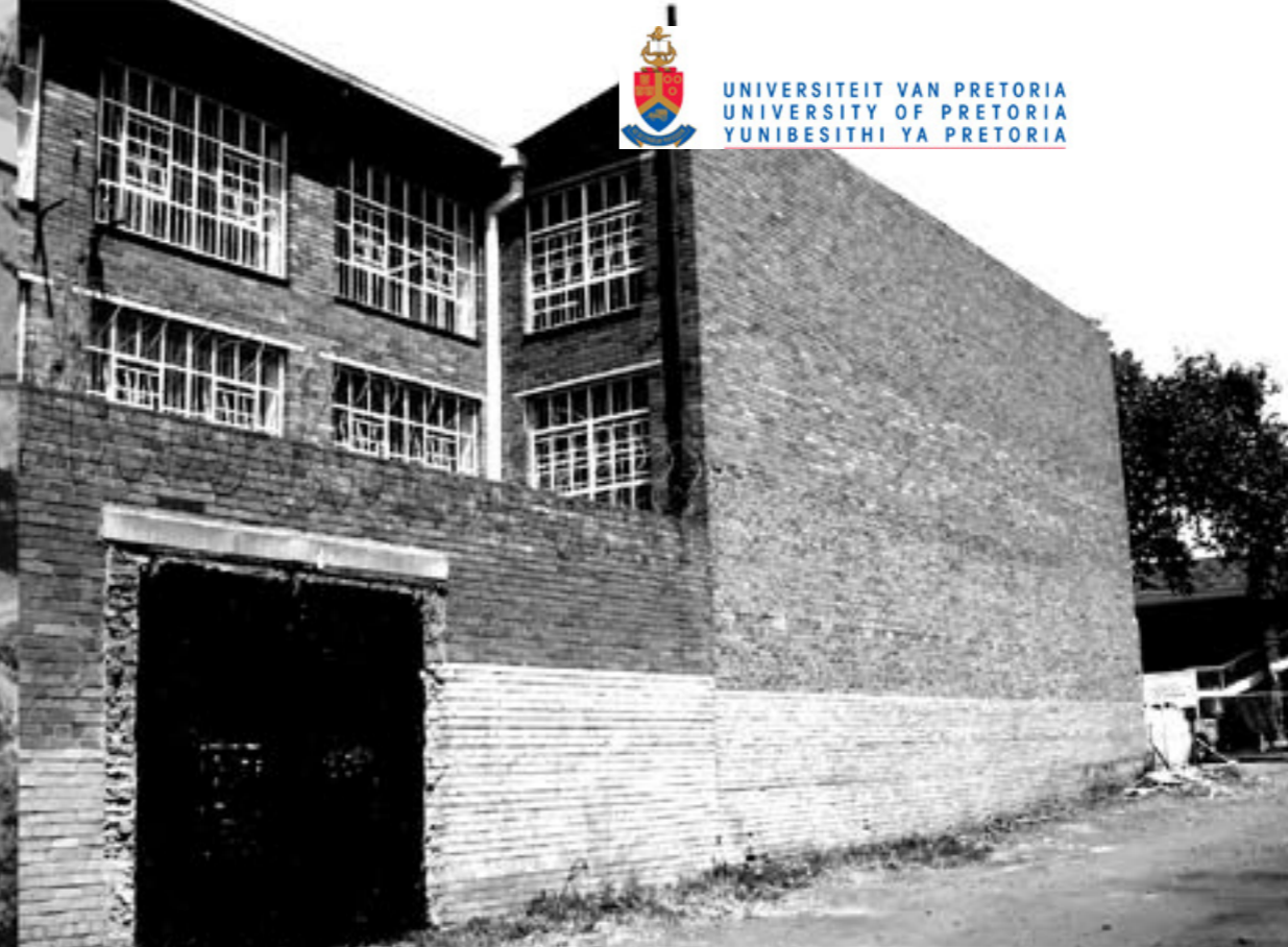
a. The building on the northern corner of the city block is three storeys high and constructed from brick masonry. It has office space on the first and second floors and retail space on the ground floor. Large parts of the building have been demolished and some parts even destroyed by fire. It is currently standing vacant and is of low economic value.
