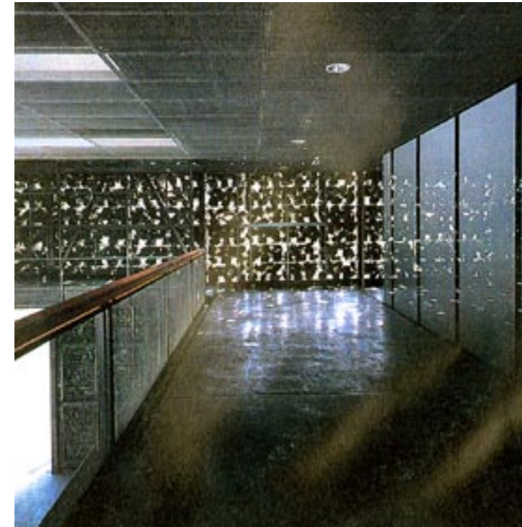
Fig.59: Interior view of the Dominus Winery showing sunlight penetrating the gabion wall.
