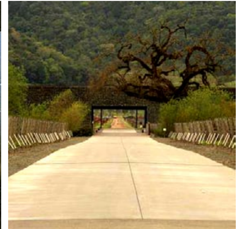
Fig.60: Exterior view of the Dominus Winery showing an undercover walkway puncturing through the building
