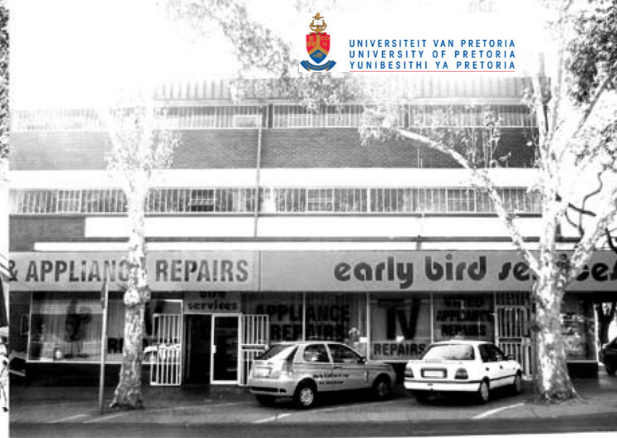
Fig. 51: Ground floor retail and upper story offices. Offices are standing vacant.
