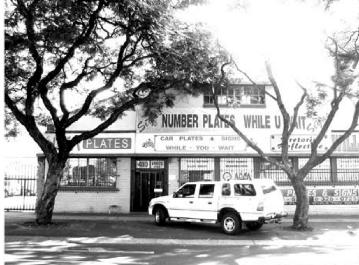
Fig. 53: Street facing side of the building.
