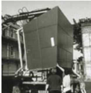
Figure 156: Installation of Bradbury St. vendor stalls.
