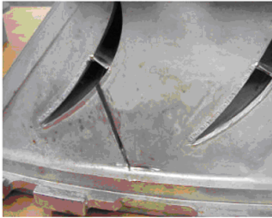
Figure 3: Ground out cracks on an X-45, W501F, Row 3 vane.
