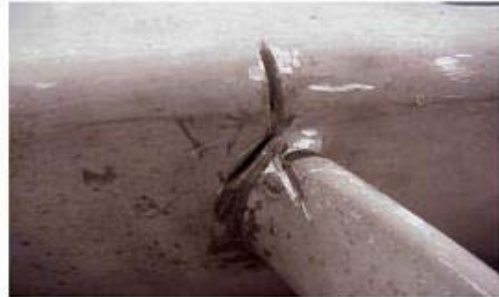
Figure 37(a) – Routed crack
