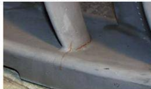
Figure 5 – Typical crack on the vane segment
