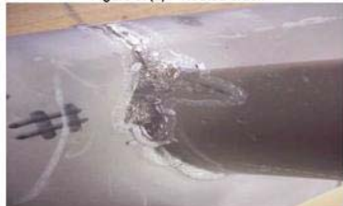
Figure 37(b) – repaired area
