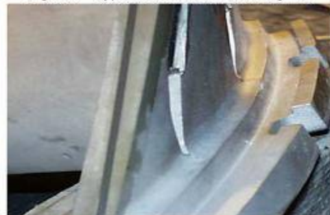
Figure 6 – Hook fit area, which needs to be restored
