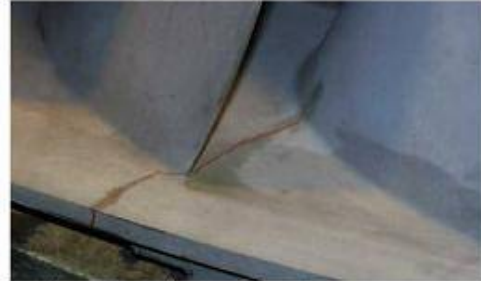
Figure 3 – Typical crack on the vane segment
