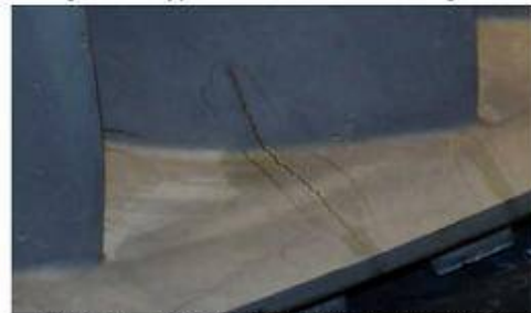
Figure 4 – Typical crack on the vane segment
