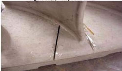
Figure 36(a) – Routed crack
