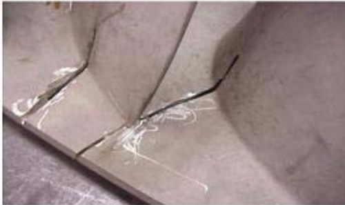
Figure 35(a) – Routed crack
