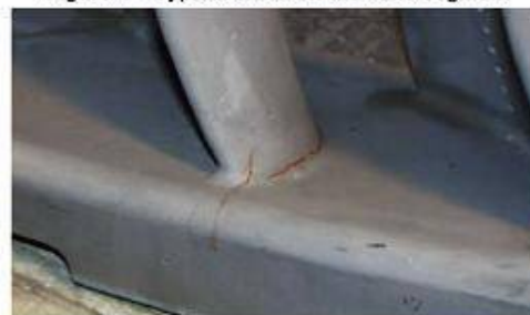
Figure 5 – Typical crack on the vane segment
