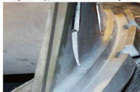
Figure 6 – Hook fit area, which needs to be restored
