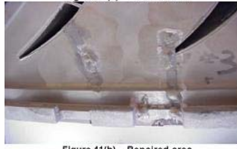
Figure 41(b) – Repaired area
