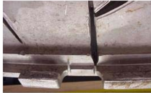
Figure 41(a) – Routed crack
