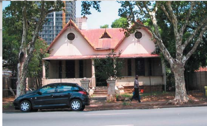
Figure 4.3.7 : The residential heritage building
