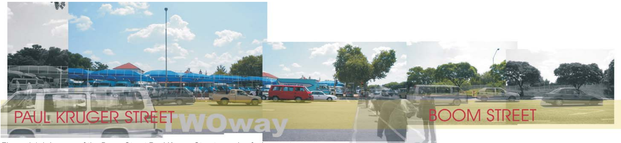
Figure 4.1.4: Images of the Boom Street Paul Kruger Street crossing facing west
