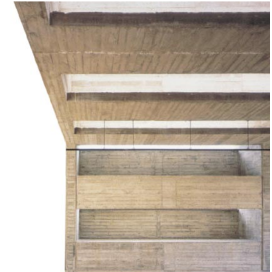
Fig. 113 Off shutter concrete wall patterned by the grain of timber shuttering planks. GPY Architectos. San Bernardo Assembly hall and workshop space, 1999-2001, Los Silos, Tenerife, Spain. (Hadid, Z. Forster, K. Sudjic, D. et al. 2005: 131)
