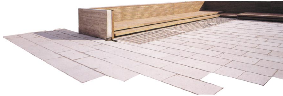
Fig. 116 Pre-cast concrete block floor. Atelier Barani, Youth Studio at the concrete art centre, 1997-1998, Moulans-Sartoux, France. (Hadid, Z. Forster, K. Sudjic, D. et al. 2005: 46 – 47)
