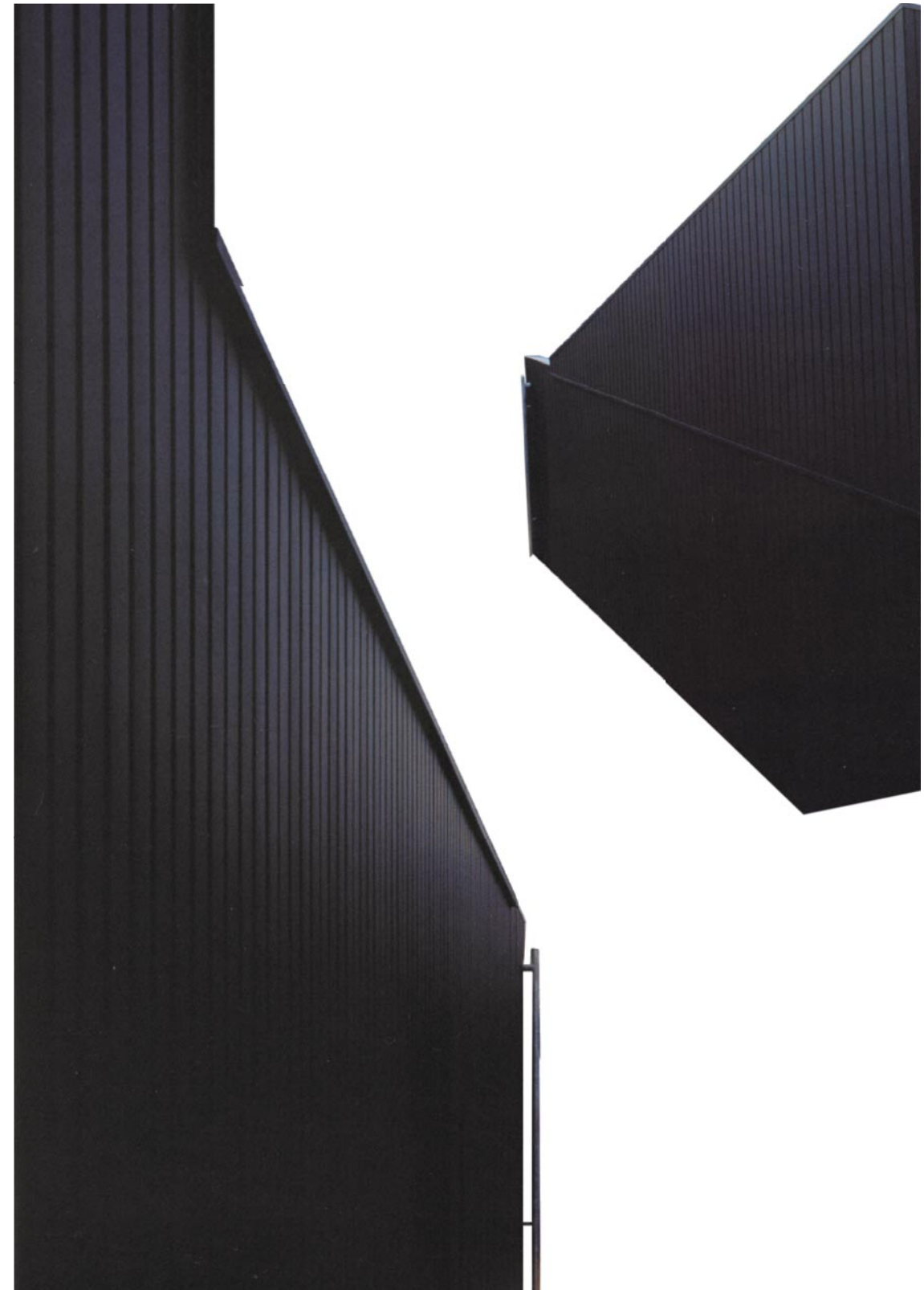
Fig 115 Powder coated black intumescent paint on steel sheeting. Waro Kishi & K. Associates, Hu Tong Private residence, 2002, western Japan. (Hadid, Z. Forster, K. Sudjic, D. et al. 2005: 398 - 399)
