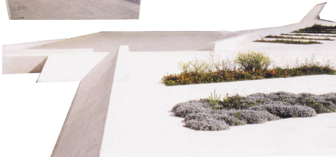
Fig. 117 Planter laid flush in concrete screed. J. Miguel Hernandes León, Murallas de Ceuta, 1992-1999, Ceuta Spanish enclave in Marocco (A. Aymonino, V. P. Mosco 2006: 48)
