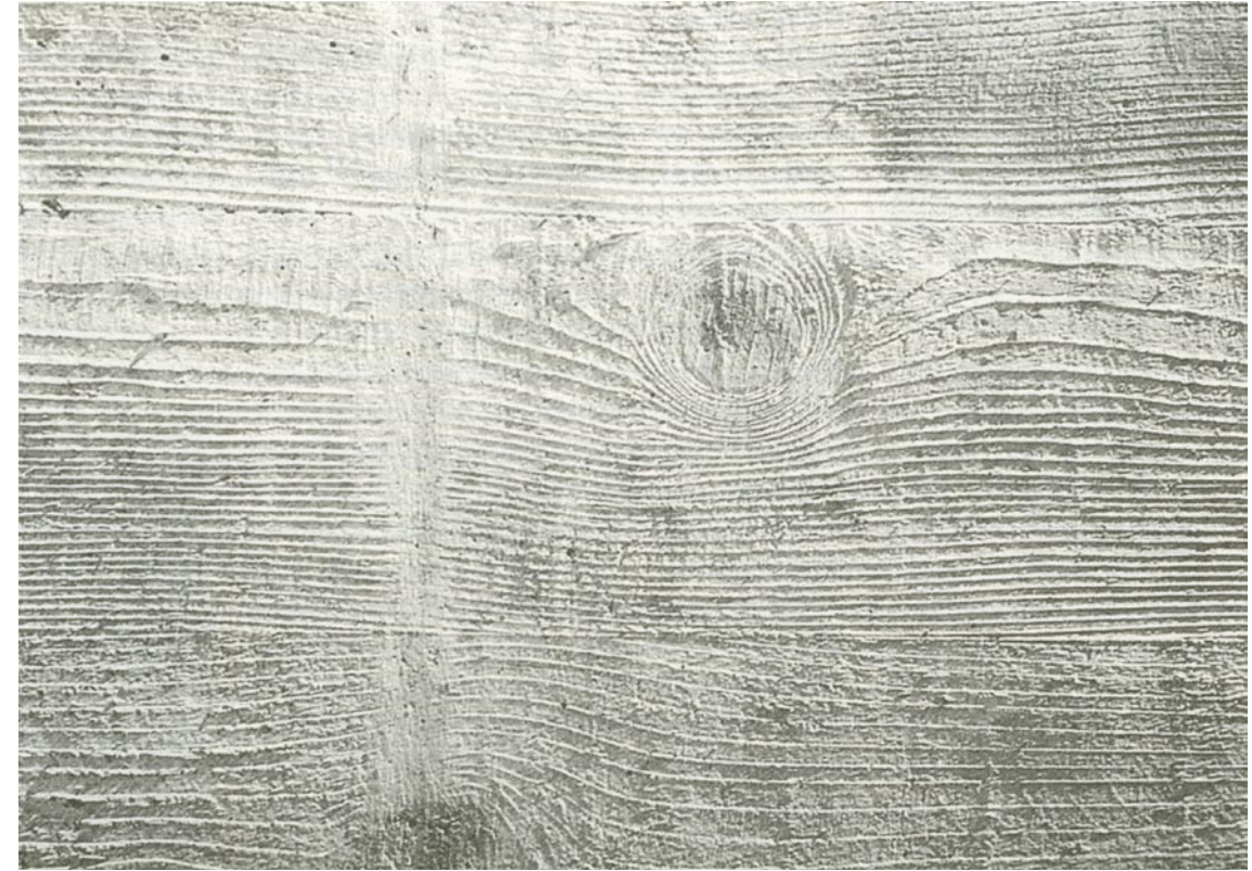
Fig. 112 Concrete texture created by rough sawn timber boards (Deplazes 2005: 57)
