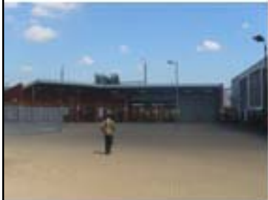
Figure 1.4.34 Bosman train station
