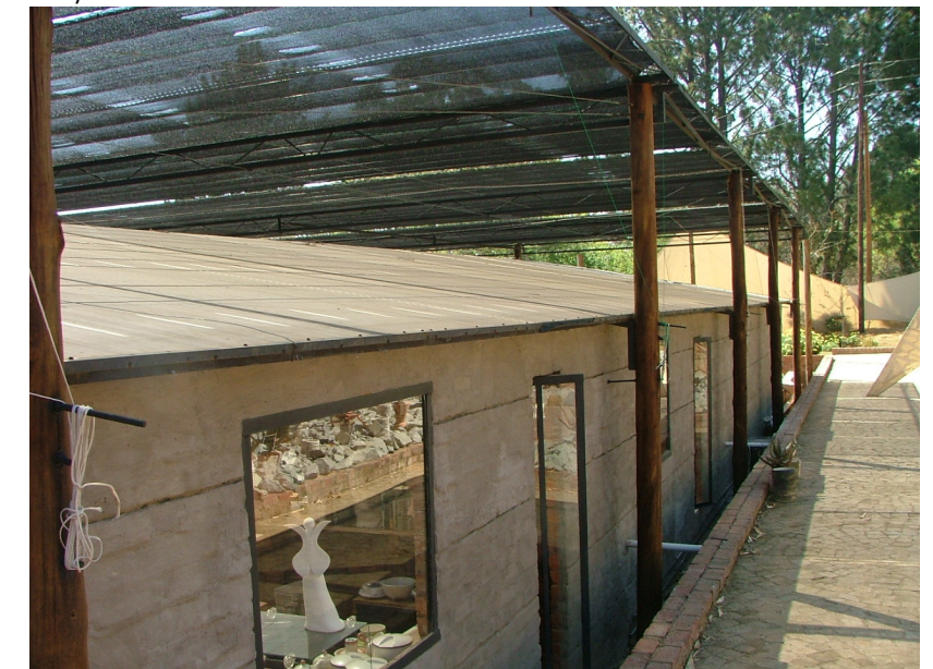
Fig 32: Purple Daisy images: ambient diffused light as a result of the roofing material. The allowance for large uninterrupted spaces, as the need for columns and supports is eliminated (Tumubweinee, 2006)
