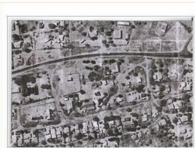
aerial view_SAUSSPOORT TOWN
